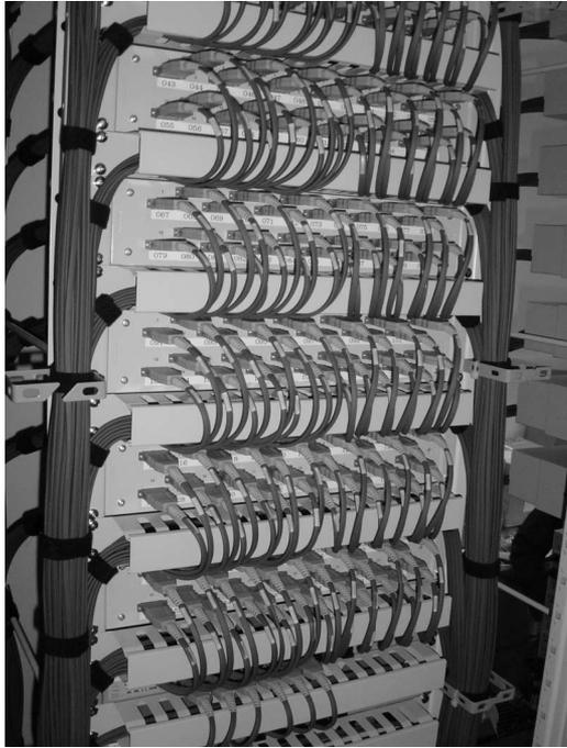
Fig. 20. Photo of a patch-panel placed in a cardiac hospital.
